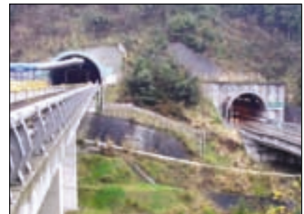
Tunnel Portal and original road tunnel (right)
