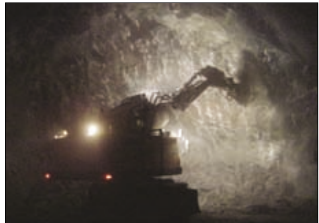
Removal of tights prior to spraying of shotcrete.
