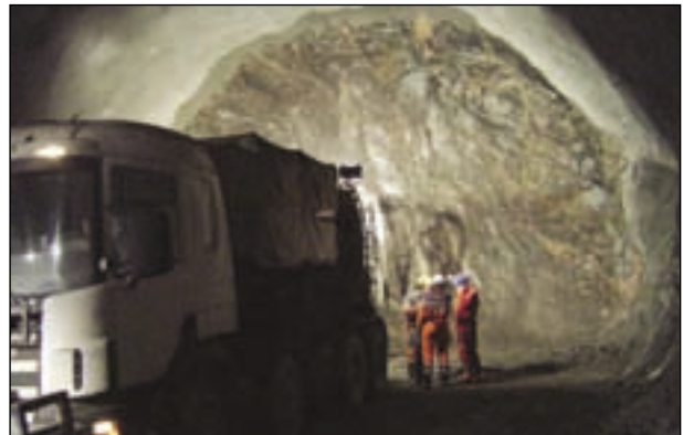
Preparation for spraying Barchip fibre shotcrete insitu.
