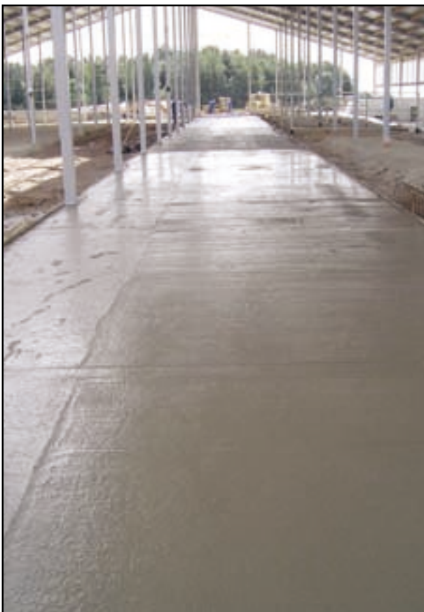
Concrete floor prior to finishing
