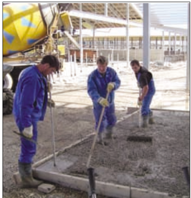
Placing Barchip reinforced concrete
