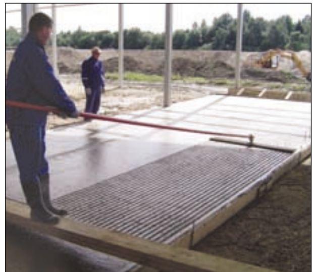
Applying the floors unique finish
