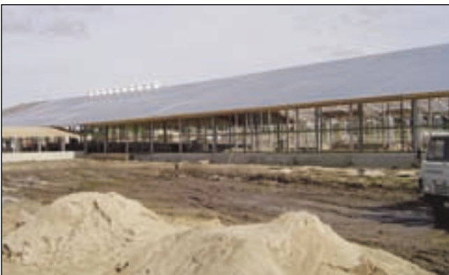
Cattle house under construction
