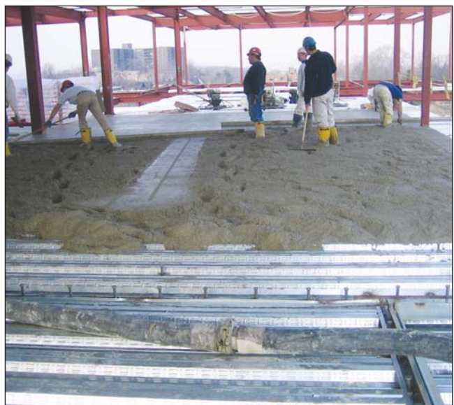
Pumping concrete to 4th floor
