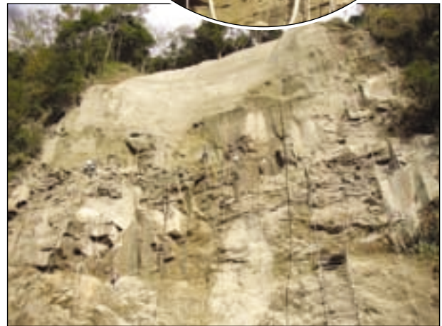
The completed upper face of the embankment
