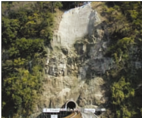
View of the embankment and the railway line approach
