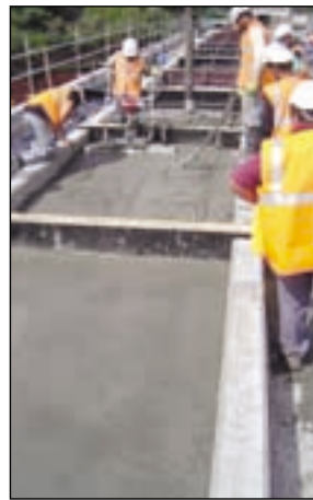
Pouring and finishing of the track slab.
