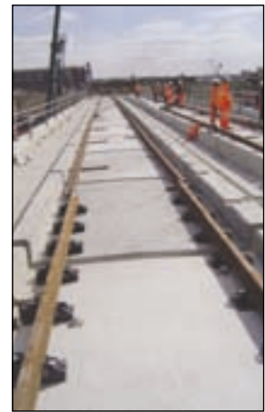
Completed track ready for installation of track rail.
