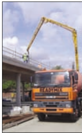
Barchip reinforced concrete is pumped up onto the elevated railway.
